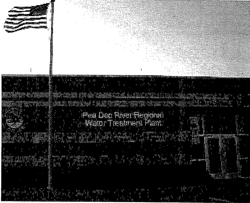
Figure 6-28. City of Florence Surface Water Treatment Plant.
